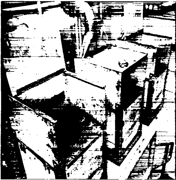
Fig. 19. Early induction-heated graphitizing furnaces.
